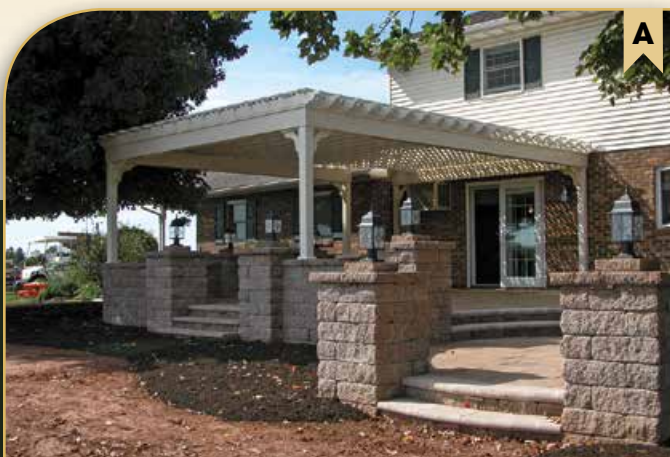
A - CUSTOM VINYL TRADITIONAL Glu-Lam Beam Made to Span 22' Opening & Custom Fit Corner of House
